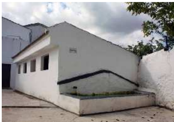
Pilar -Lavadero de la Aldea (B. Montes, mayo 2010)
